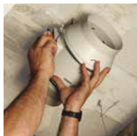
Place the impeller and motor.
