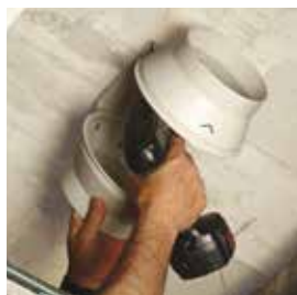
Fix the support bracket.
