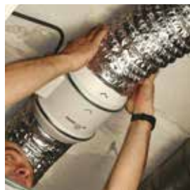
Connect the ducts.
