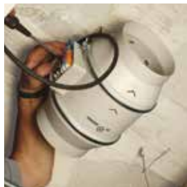
Carry out the wiring connections.
